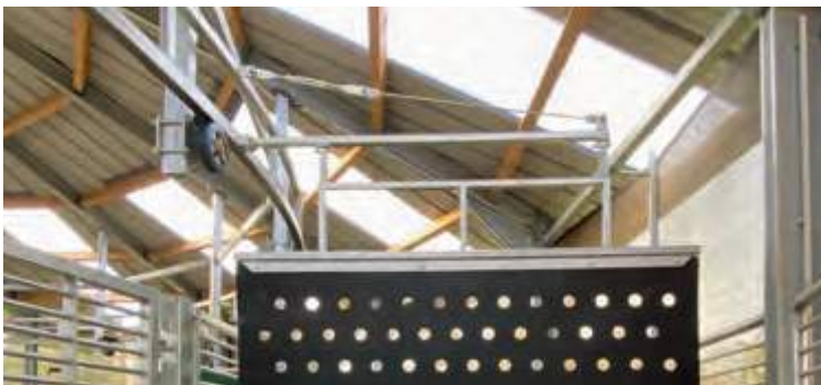
Stable guidance for the rotating gates
