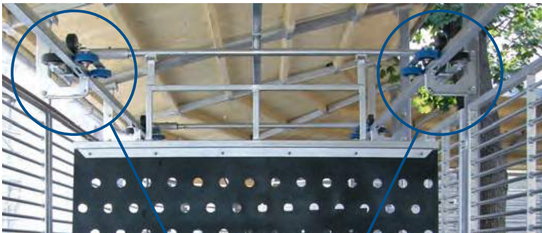
Double track to improve safety and stability
